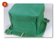
Place canopy above aperture, with flaps turned outwards flat against the ceiling surface and overlapped at the corners.
