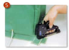
Secure canopy to ceiling with stainless steel staples of a minimum 12mm length and wire size 20 gauge (0.5 x 1.25mm) at 80mm centres along the four flaps.
